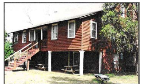
The John Ford House, constructed 208 years ago, is the oldest remaining residence on the Pearl River.
